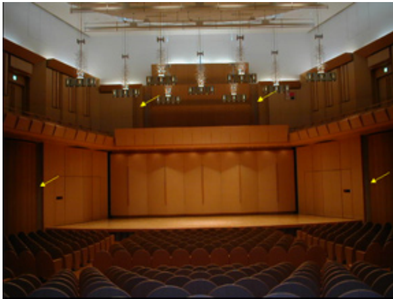
Figure 20. The line arrays are so well hidden in this facility they are impossible to locate. (They are mounted to each side of the stage and next to the pipe organ for the balcony as shown by the arrows.) In this auditorium, both the unobtrusiveness and speech intelligibility performance of the arrays made them a clear winner over a conventional approach.
