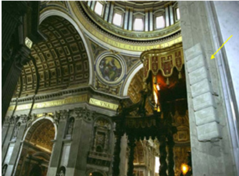
Figure 17. One of the custom made line arrays used in St. Peter's Basilica is shown (arrow).
