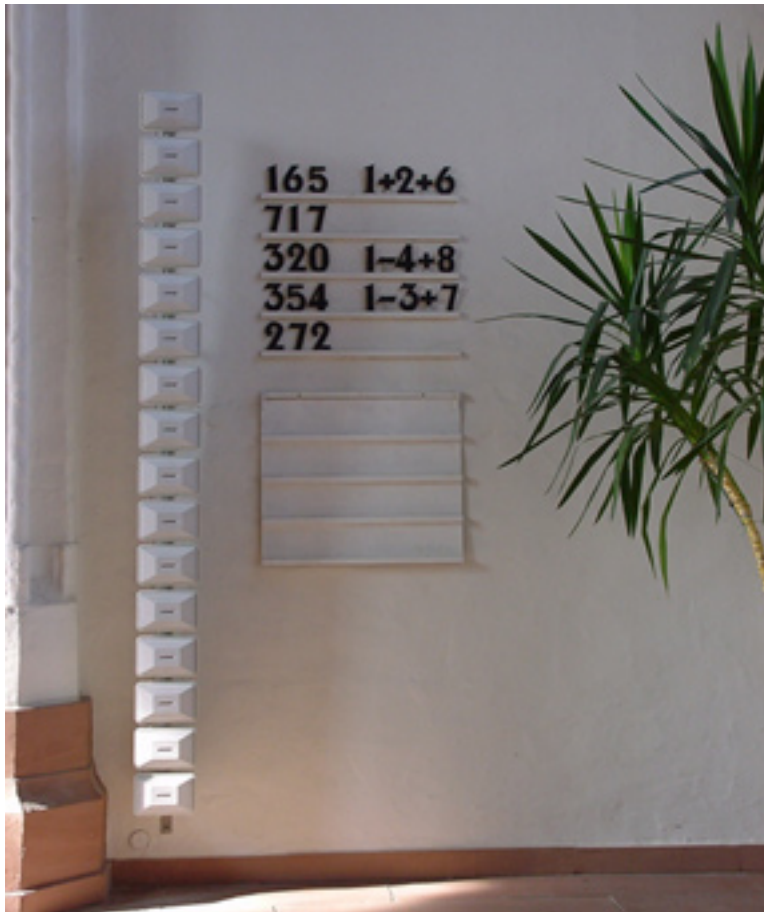
Figure 22. A close up of the line array is shown. It is made from sixteen Bose Model 101s.
